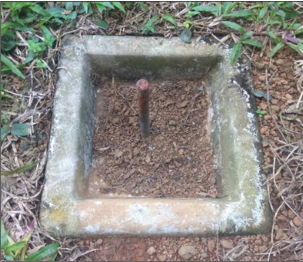
Figure 5. One of the untreated earthing electrodes (EE-3)
