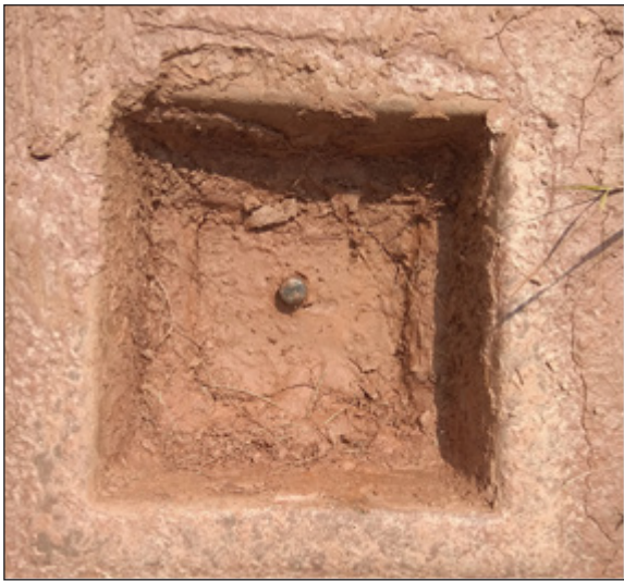
Figure 7. An industrial earth resistance reduction agent earthing (treated earthing)
